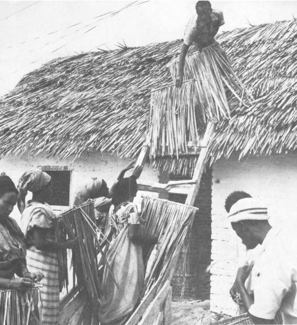
Townspeople putting a thatched roof on a new house Courtesy United States International Communication Agency
